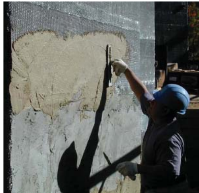
Fig. 1B - Applying scratch coat of mortar
